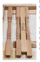
by screwing the 2 ¼" screws through the sub-rail and into the spindle. For larger spindles such as 2 ½" or 3 ½", two screws in each spindle/baluster end should be used. Many find it easiest to make a spacer block to place between spindles as they are screwed into place.
