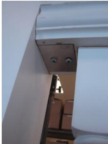
Photo No. 5 Top Rail - Bracket - Post Connection
